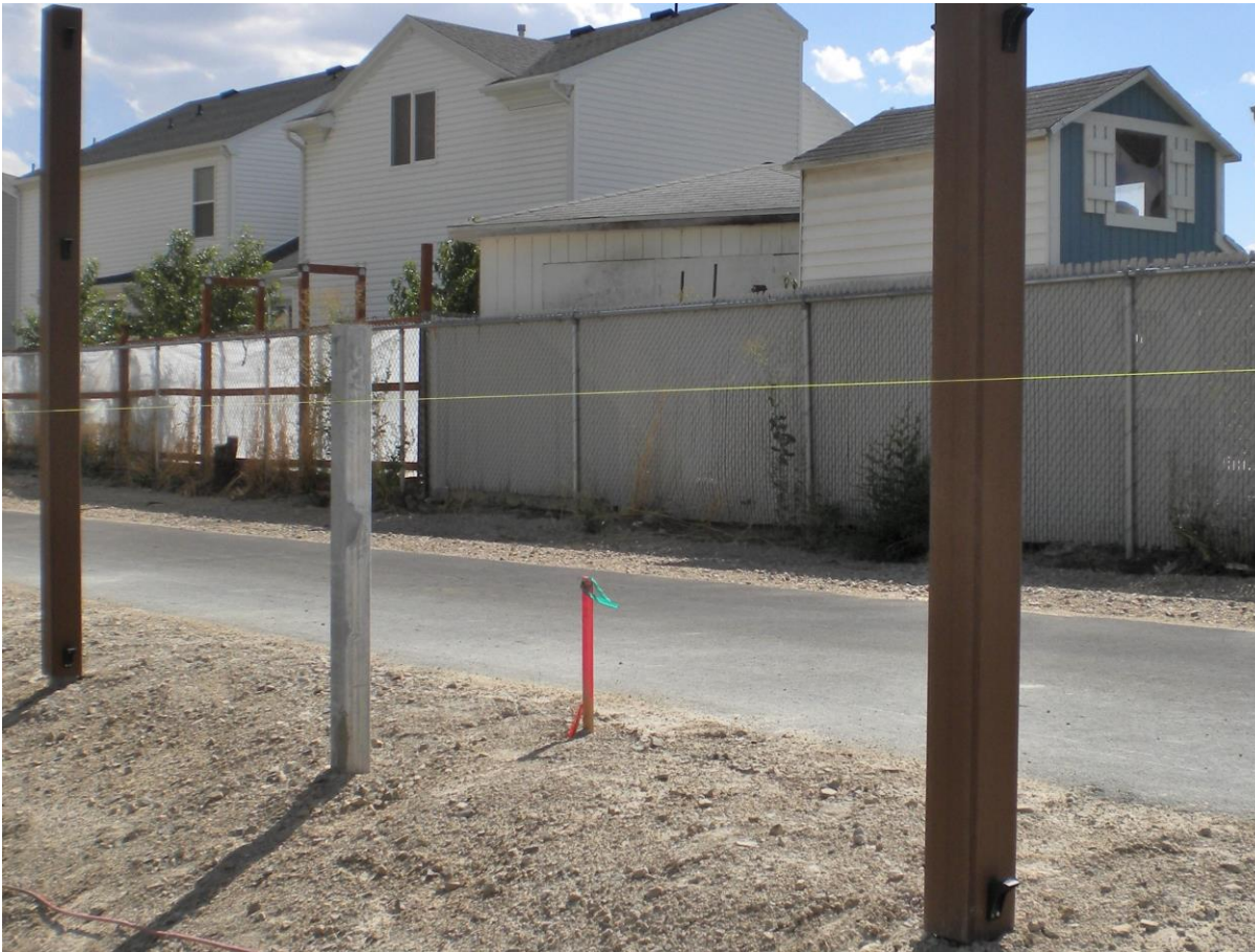
5"x5" Composite Post sleeve over Steel Post Stiffener
